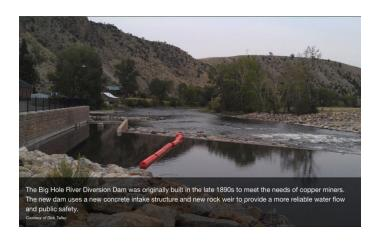
The old structure was removed and replaced with a new concrete intake structure and a new rock weir. The new intake structure now provides a more reliable water flow from the river to the existing pump house. The newly constructed dam also took into account recreational use and boater safety, creating a boat and fish passage channel. Most importantly, the dam has provided Butte the security of drawing water from the Big Hole River for years to come.
