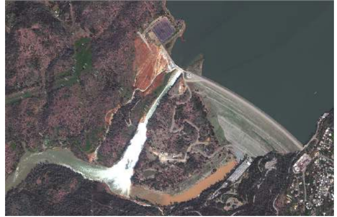
The two spillways of the Oroville Dam during the February 2017 overflow (main at right, auxiliary at left). Photo: DigitalGlobe
